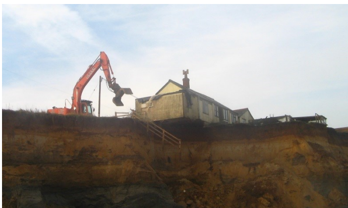
Figure 12: A property at risk of coastal erosion being demolished (image courtesy of North Norfolk District Council)
